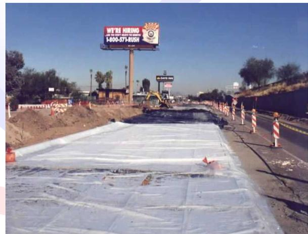
Figure 1. Pavement protected with polyethylene sheets.
