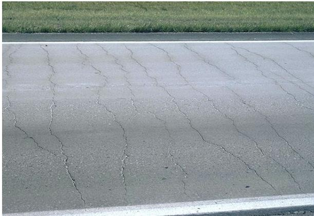
Excessive thermal cracking is often due to high temperature differentials, excessive subbase friction, aggregates with high coefficients of thermal expansion/contraction, or a combination of the above.
